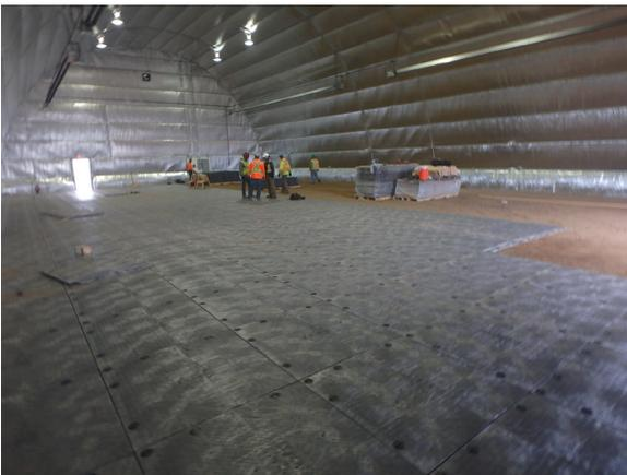
The plastic Matrax matting system is a perfect solution to solve this problem and avoid an expensive concrete floor. The extremely low temperatures were beyond the capabilities of the standard plastic products so Matrax added plastomers (materials designed to alter the crystallinity of the HPDE) to the formula and manufactured flooring panels specifically for this Suncor Energy application. The modification of the HPDE with plastomers resulted in better
