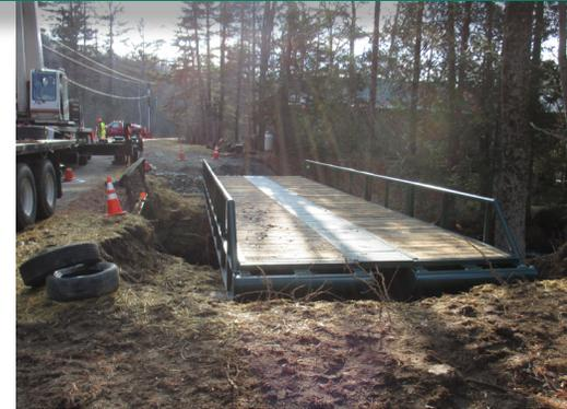
Immediate action was required as traffic was already restricted to one lane and winter weather was preventing any repairs until spring. It was at this time that Highway Department Superintendent, Dan Hitchcock, engaged Matrax Inc. for a temporary bridge solution. A portable temporary hinged bridge measuring 50 feet long was recommended by Matrax to be a suitable quick-fix for the winter months leading up to and during the Garnet Lake Road Bridge repair.
