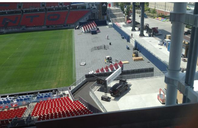
Given this heavy equipment configuration, it was determined that approximately 24,000 square feet of drivable turf protection was needed for the end zone areas in which the temporary stadium seating, VIP guests, forklifts, vendor stands, and additional traffic would need to traverse the sensitive turf. BMO Field contacted Matrax looking for an efficient solution.
